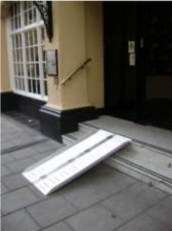
**Assistance is likely to be required to use the ramp as it has a gradient of 1:4.** It is 1500mm long and 730mm wide. This is a temporary solution.
