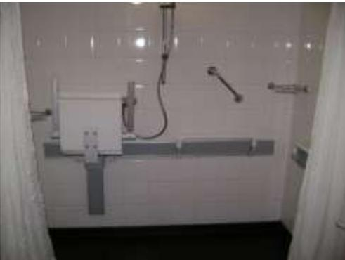
There is lateral transfer to the adjustable height shower seat of 1260mm to the right. The seat is fitted with integral fold down armrests.
