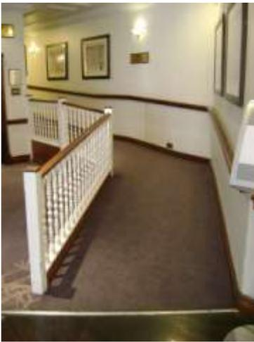
Access to the Clifton Room, the public WCs and Marlow's is via an internal ramped route which is a minimum of 1400mm wide. This series of ramps has gradients of 1:12 – 1:16 and are 2.5m, 2m and 6m long with resting places.
