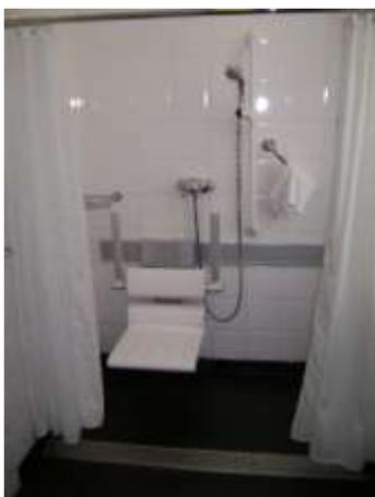
There is lateral transfer to the adjustable height shower seat of 900mm to the right. The seat is fitted with integral fold down armrests.
