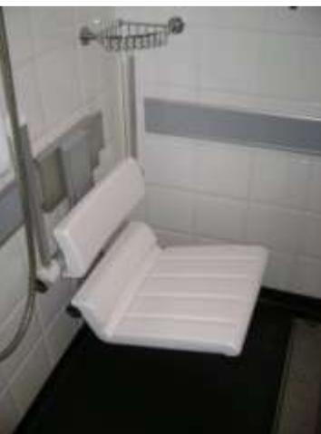
There is lateral transfer to the adjustable height shower seat of 1500mm to the left. The seat is fitted with integral fold down armrests.
