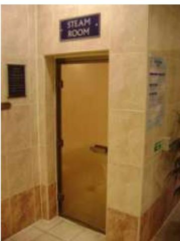
The Steam Room has a 650mm clear opening door with a 50mm step.
